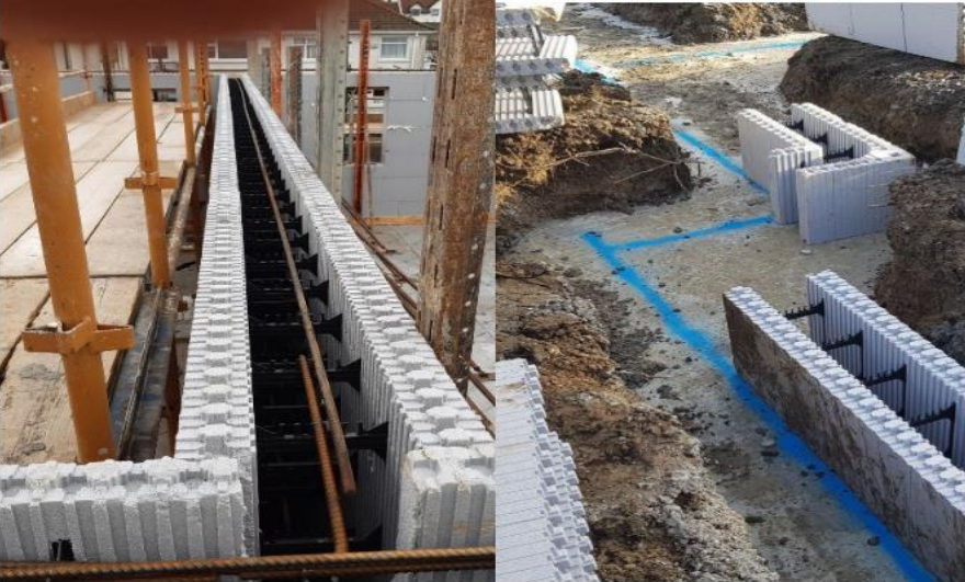
Figure 1: ICF Construction
