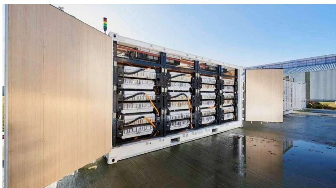
Figure 1: BESS comprised of EV batteries
