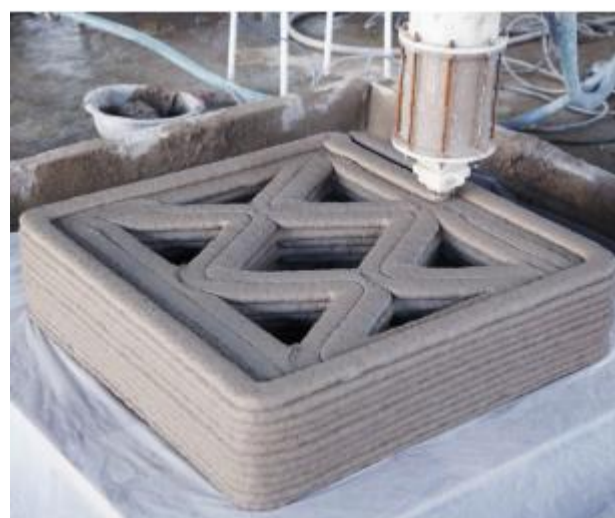
Figure 1 concrete printing of a section of a pedestrian bridge
