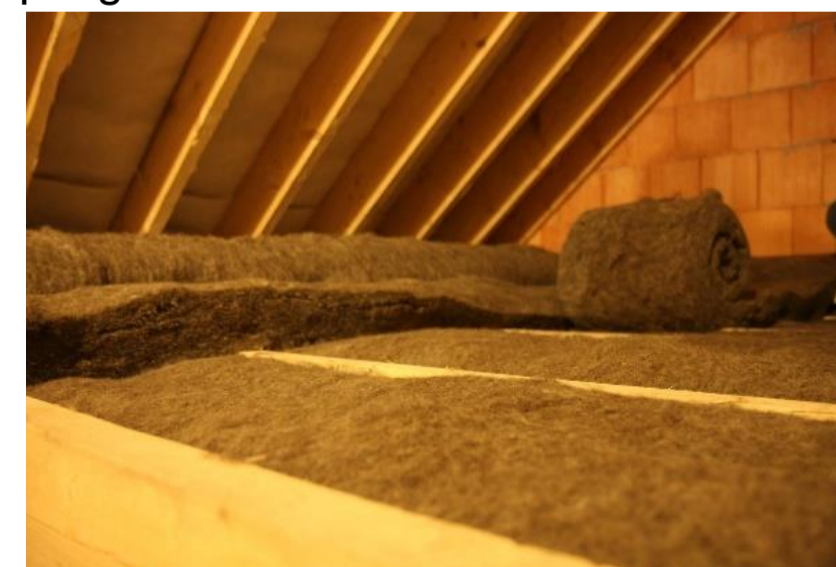
Figure 4 Sheep wool Insulation in attic
