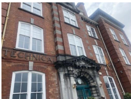
Iconic Education and Training Board Building in Limerick: the test bed for DECO2 in Ireland
